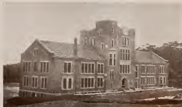
Underwood Hall, Rear Elevation
